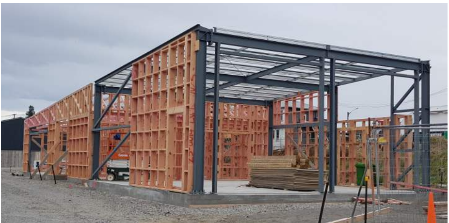
The frame is up for Taihape's new St John's Centre
