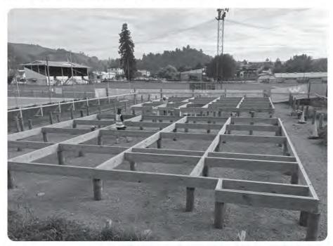
Thanks to the recent clear weather Ngā Awa Block (Taihape Amenities) project continues to track along nicely. Piling has now been completed and the structure has been built for the floor panels. You can head along to the tennis and netball courts to view the progress from outside the barrier.
